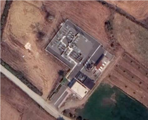
Figure 5 - The existing Kajan substation
